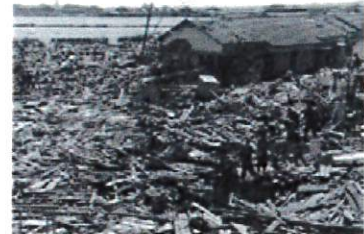
Damage by the Isewan Typhoon (photo provided by Aichi Prefectural Government)
