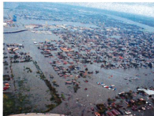
Damage caused by Hurricane Katrina
