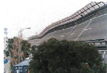
Destructed viaduct of the Hanshin Expressway (photo provided by Kobe City)
